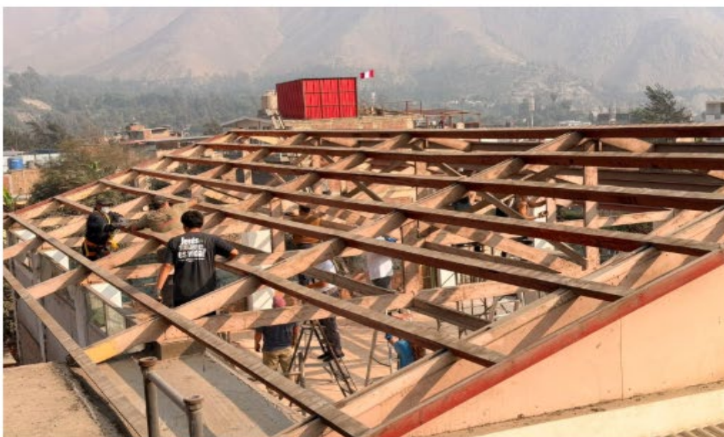
The group helped us remove the old roof from the third-floor auditorium and install a new one. This is where we hold our larger conferences and ministry events.
